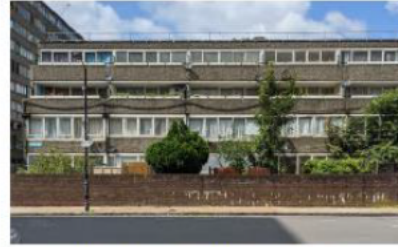
1. A view north from Kinglake Street to the existing buildings
